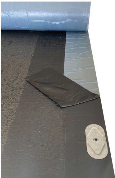
Place the fastening under the selvedge
